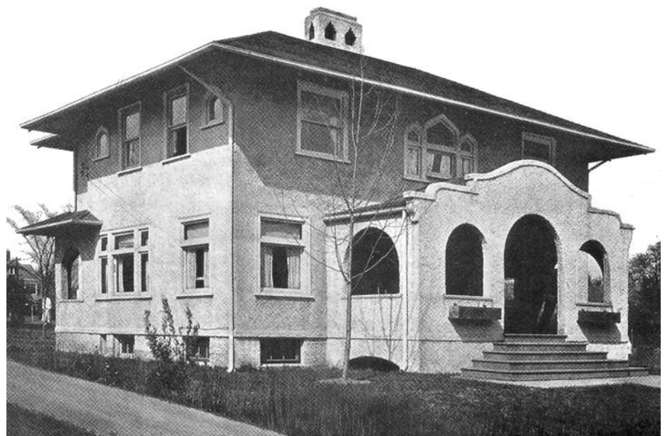
The Dudley and Hilda Van Antwerp residence (1902). Concrete Country Residences , Atlas Portland Cement Co., 1906.
